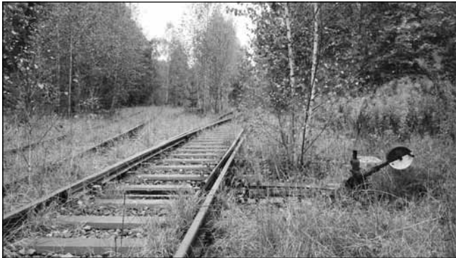
Foto: Station C23
